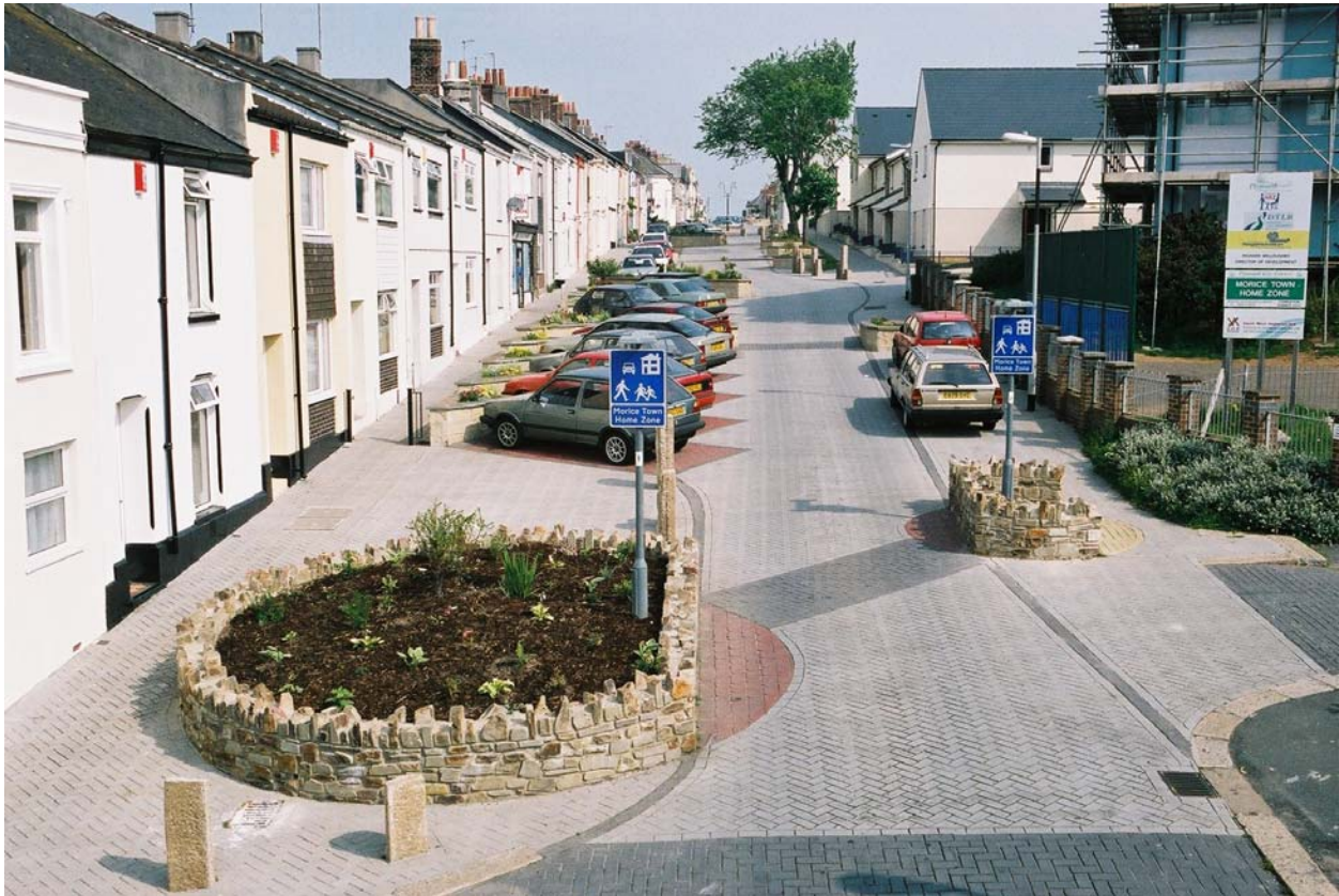
Figure 3: A British Home Zone uses decorative planters to narrow the roadway
