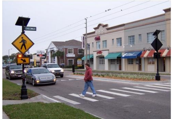
Exhibit 15 Rectangular Rapid Flashing Beacon
