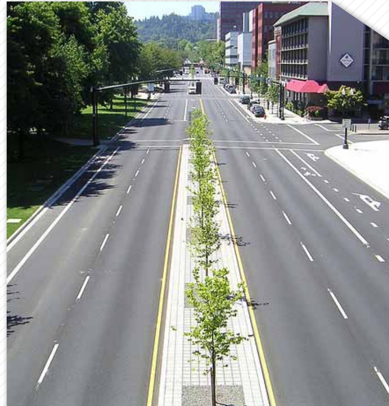
Updated in 2007, Naito Parkway in Portland, Oregon uses a planted raised median to restrict turn movements at any location that is not a signalized intersection
