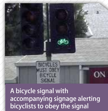
A bicycle signal in use in San Luis Obispo keeps motorists and bicyclists separated in time
